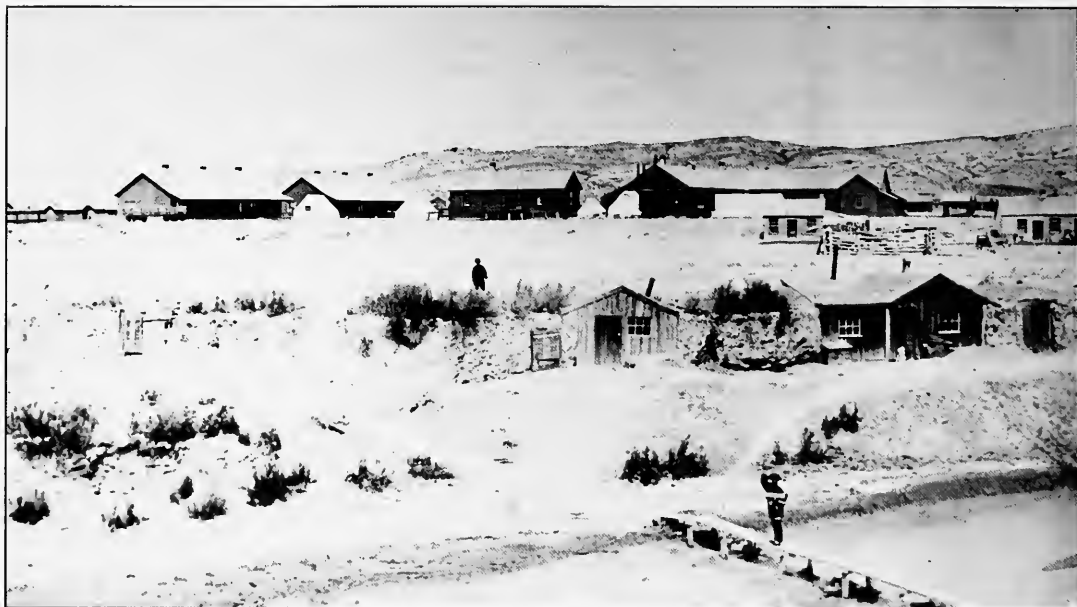
Photograph taken of Camp Pilot Butte from southwest bank of Bitter Creek. Buildings (left to right) are Officers Quarters, Quartermaster Warehouse, and Enlisted Barracks. Note freight car on siding and dugout houses in the bank of Bitter Creek.
