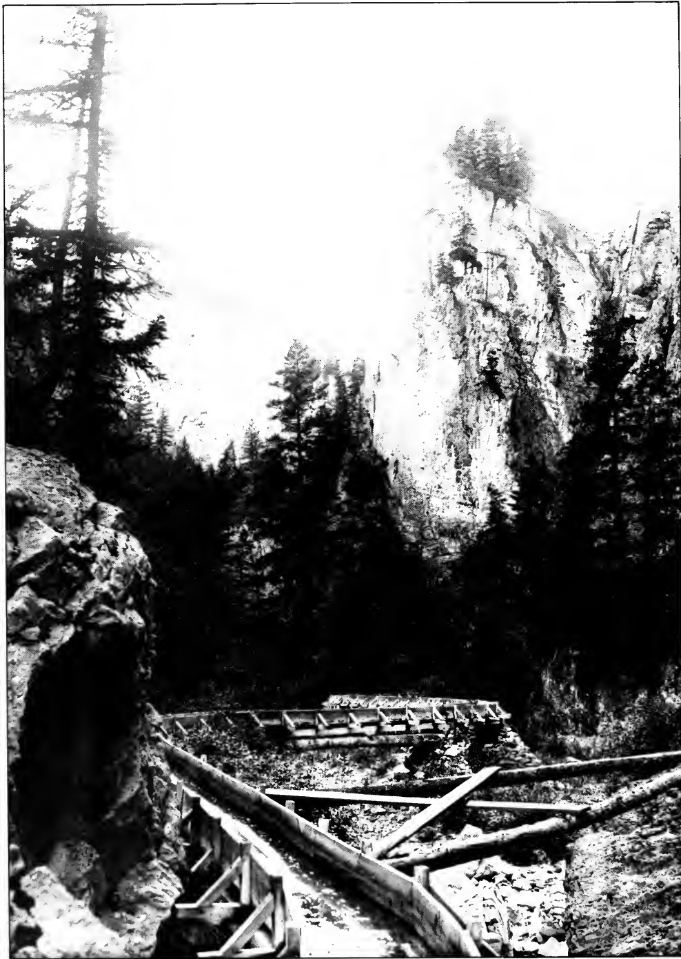
Irrigation system in Lodge Pole Canyon on the Fort Belknap Reservation.
