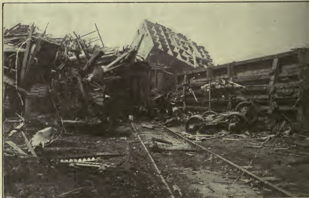
ON THE C.P.R. MAIN LINE.—The huge elevator was, with other buildings, blown right across the tracks.
