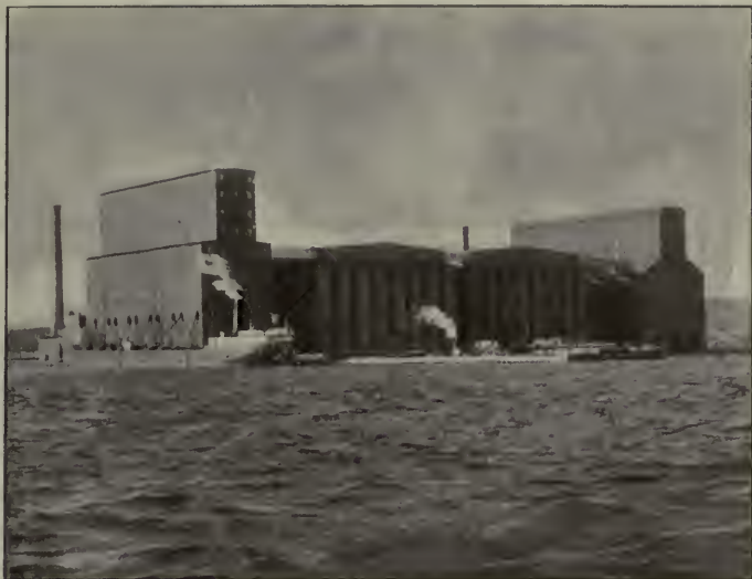
How the Railways try to keep up with the Western Grain-grower.— This is the grain elevator of the C.N.R. at Port Arthur, the largest in the world. Capacity 7,500,000 bushels. Sir Donald Mann recently stated that the capacity of this elevator will be increased to 24,000,000 bushels.
