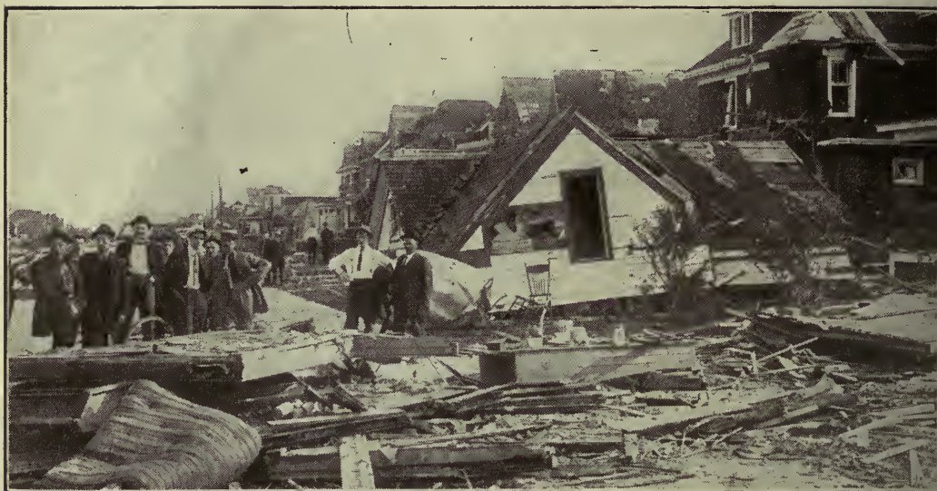
This house, with the chairs on the verandah, was carried clean across the street. The four residents were uninjured.
