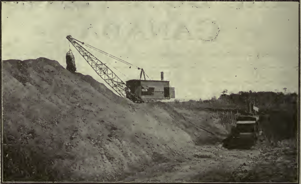
Tofield, Alberta—Steam Shovels in Operation. Lower Shovel on Coal.
