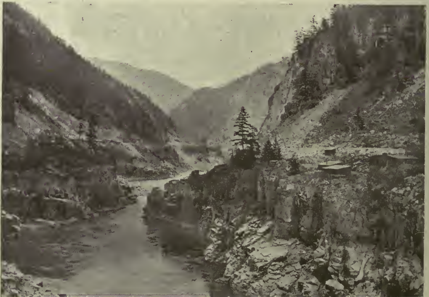
Hell's Gate, Fraser River, B.C. Engineers' Camp of the Canadian Northern Pacific on the right.
