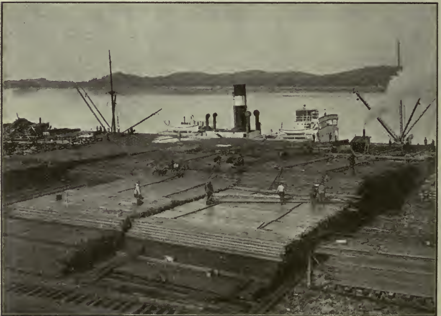
Unloading Steel at Prince Rupert for the Grand Trunk Pacific Railway.
