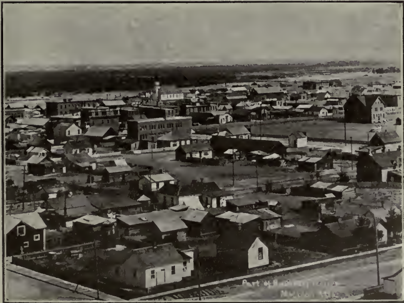
A View of Macleod—the Alberta town that is growing by leaps and bounds. Where only a few years ago small shacks existed, to-day there are substantial buildings that would do credit to any city.
