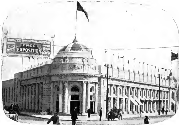
HEADQUARTERS OF THE WINNIPEG INDUSTRIAL BUREAU
