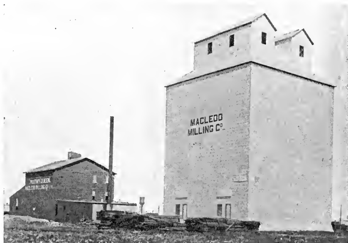
The Largest Grain Elevator West of the Great Lakes.
