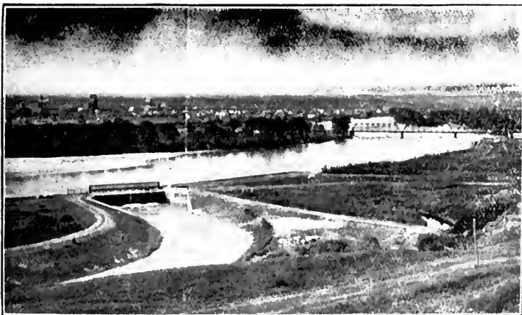
Headgates of the Irrigation System of the C.P.R., near Calgary, where 3,000,000 acres are being irrigated and sold to settlers.
