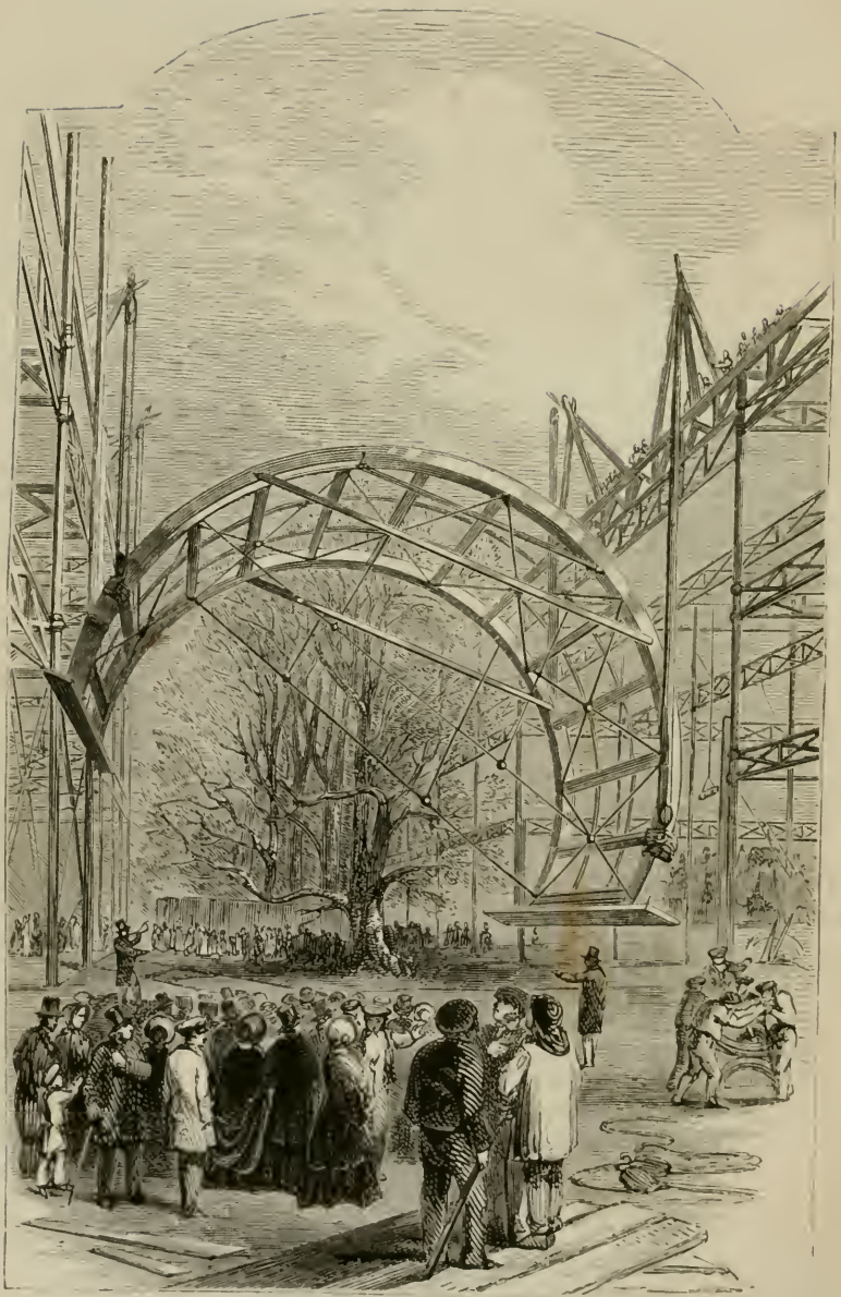
Hoisting the Ribs for the Transept Roof.
