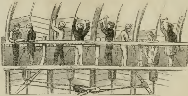
STAGE FOR GLAZING THE ROOF OF TRANSEPT.
