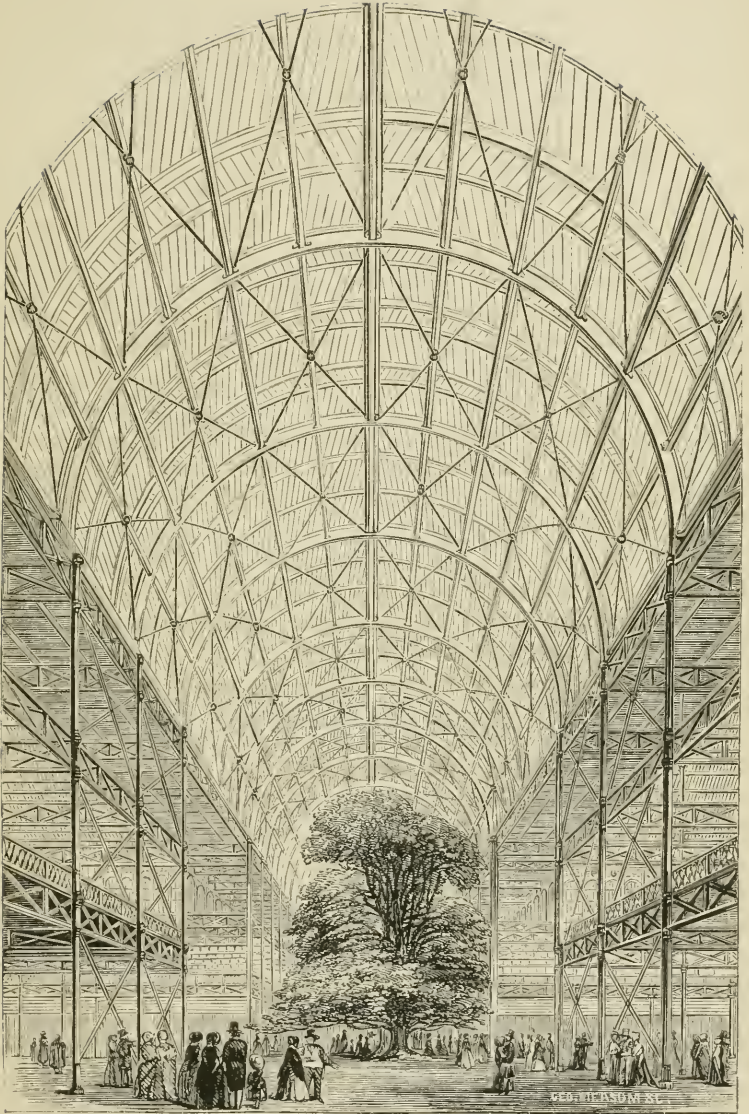
View of the Interior of the Transept.
