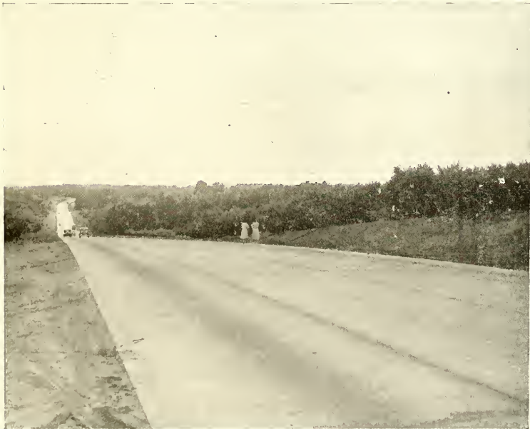
Scene on the Famous Wilkinson Boulevard (U. S. No. 29) Leading East from Gastonia, Sixty Feet Wide, Four Traffic Lanes, Carrying the Heaviest Traffic of Any Highway in the State of North Carolina
