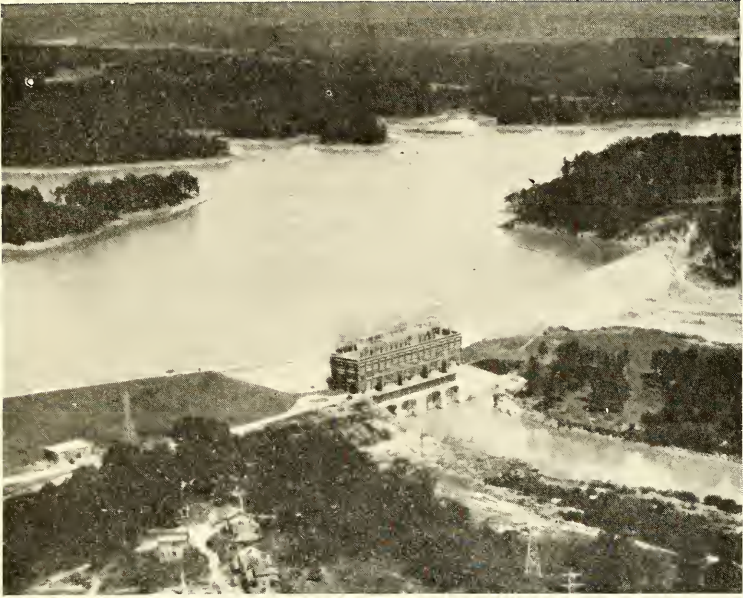
Hydro-Electric Power Plant
