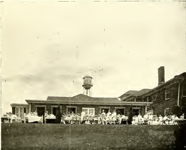
Partial View of North Carolina Orthopedic Hospital
