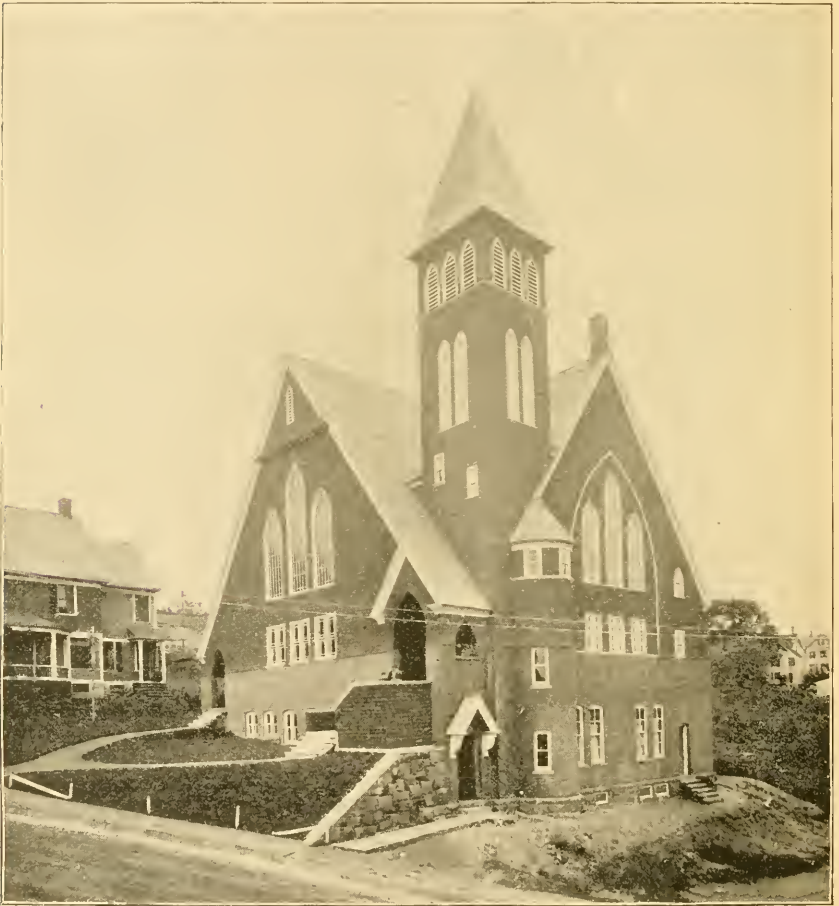
THIRD CONGREGATIONAL CHURCH, WATERBURY, CONN.
