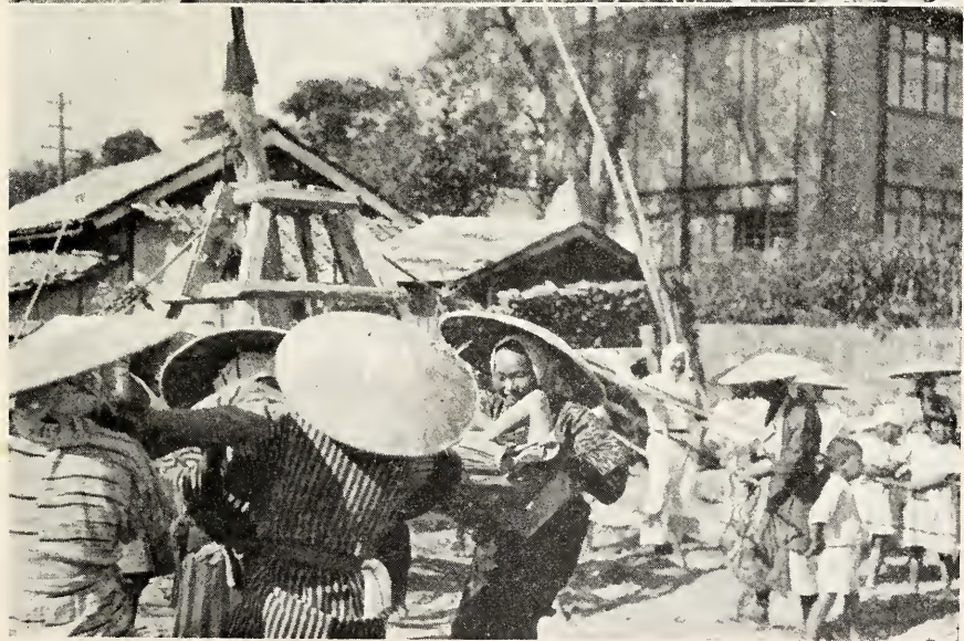
FIG. 8 ( top ) Foundation Pounding (Dotsuki).
