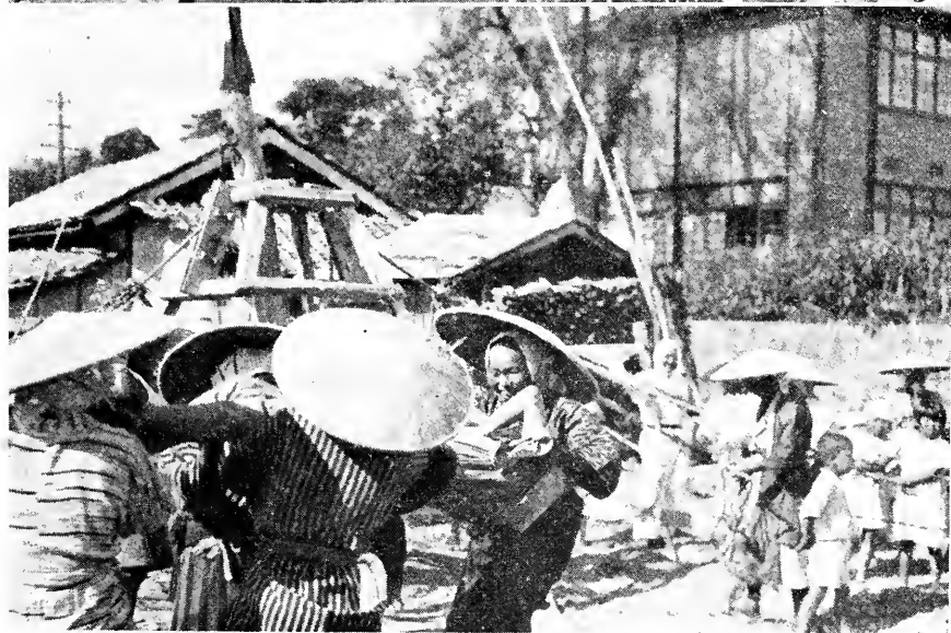
FIG. 8 ( top ) Foundation Pounding (Dotsuki).
