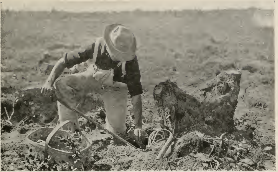
Placing One-Half a Pound of Dynamite
