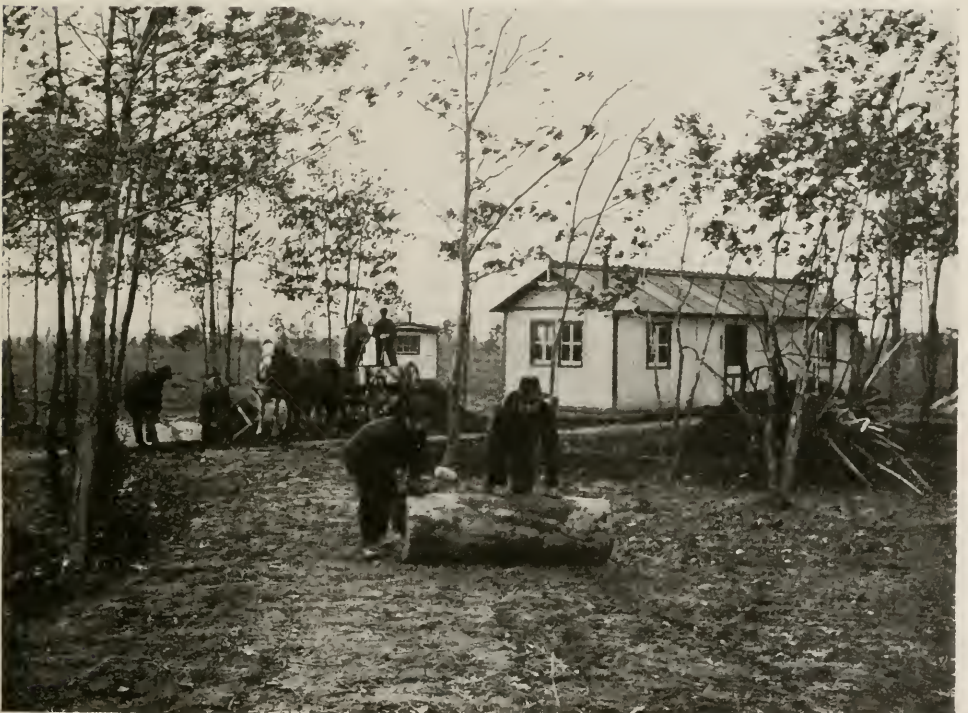
The Well-Drillers' Drop-Weight Served as a Road Roller
