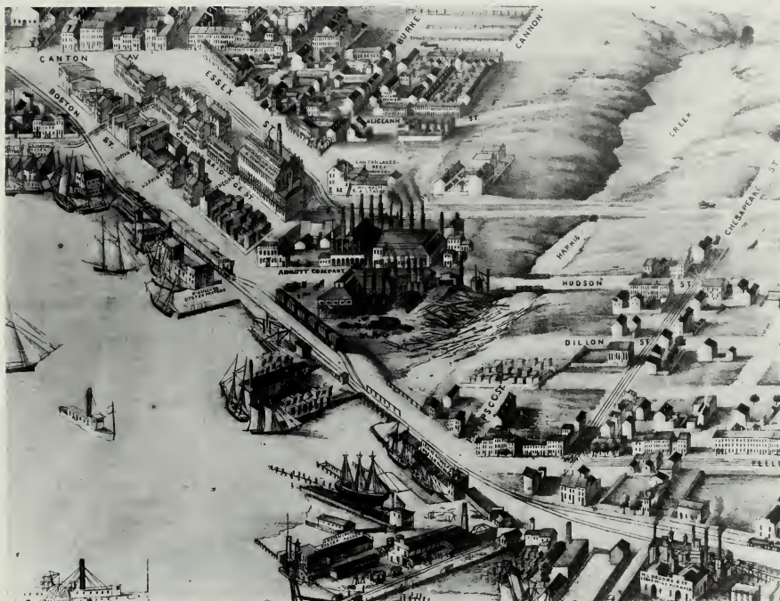
Horace Abbott's ironworks in Baltimore were one of only two large mills whose machinery could roll the thick iron plates needed to build Monitor. (The Peale Museum, Baltimore)
