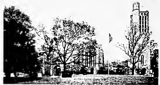
WASHINGTON MEMORIAL CHAPEL - 1914 CARILLON TOWER - 1952
