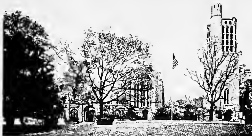
WASHINGTON MEMORIAL CHAPEL - 1914 CARILLON TOWER - 1952
