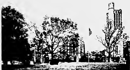
WASHINGTON MEMORIAL CHAPEL - 1914 CARILLON TOWER - 1952
