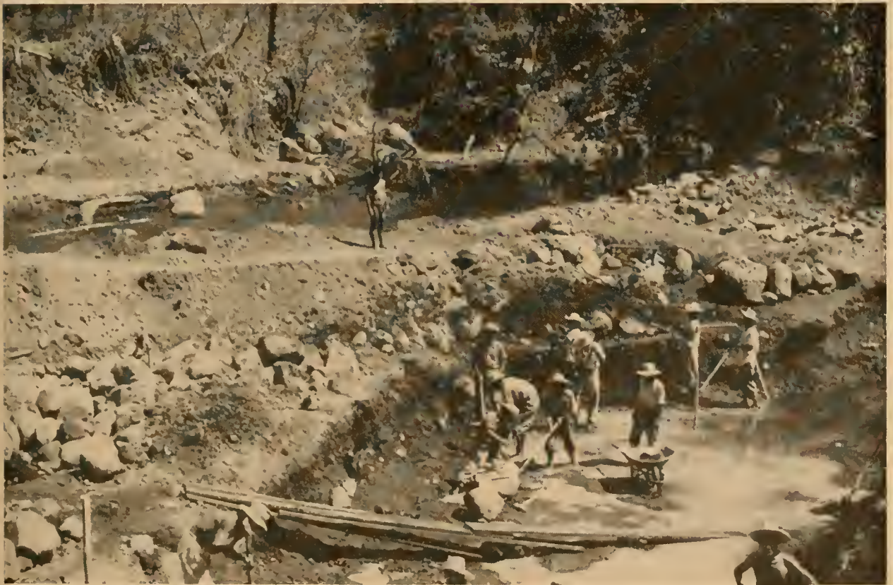
Foundations being prepared for a Pacific Slope Highway bridge across the Rio Bravo in Guatemala. The United States has earmarked $3.7 million to help complete this highway which will open coastal agricultural regions for development and help improve economic conditions in the country.
