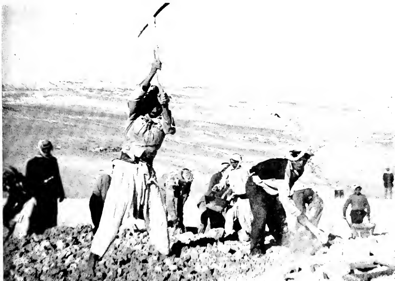
Jordanians at work on construction of an east-west highway system. Under the development assistance program, the United States is helping Jordan build more adequate road facilities to further the country's development as well as to give employment to thousands of Jordanians, including Arab refugees.
