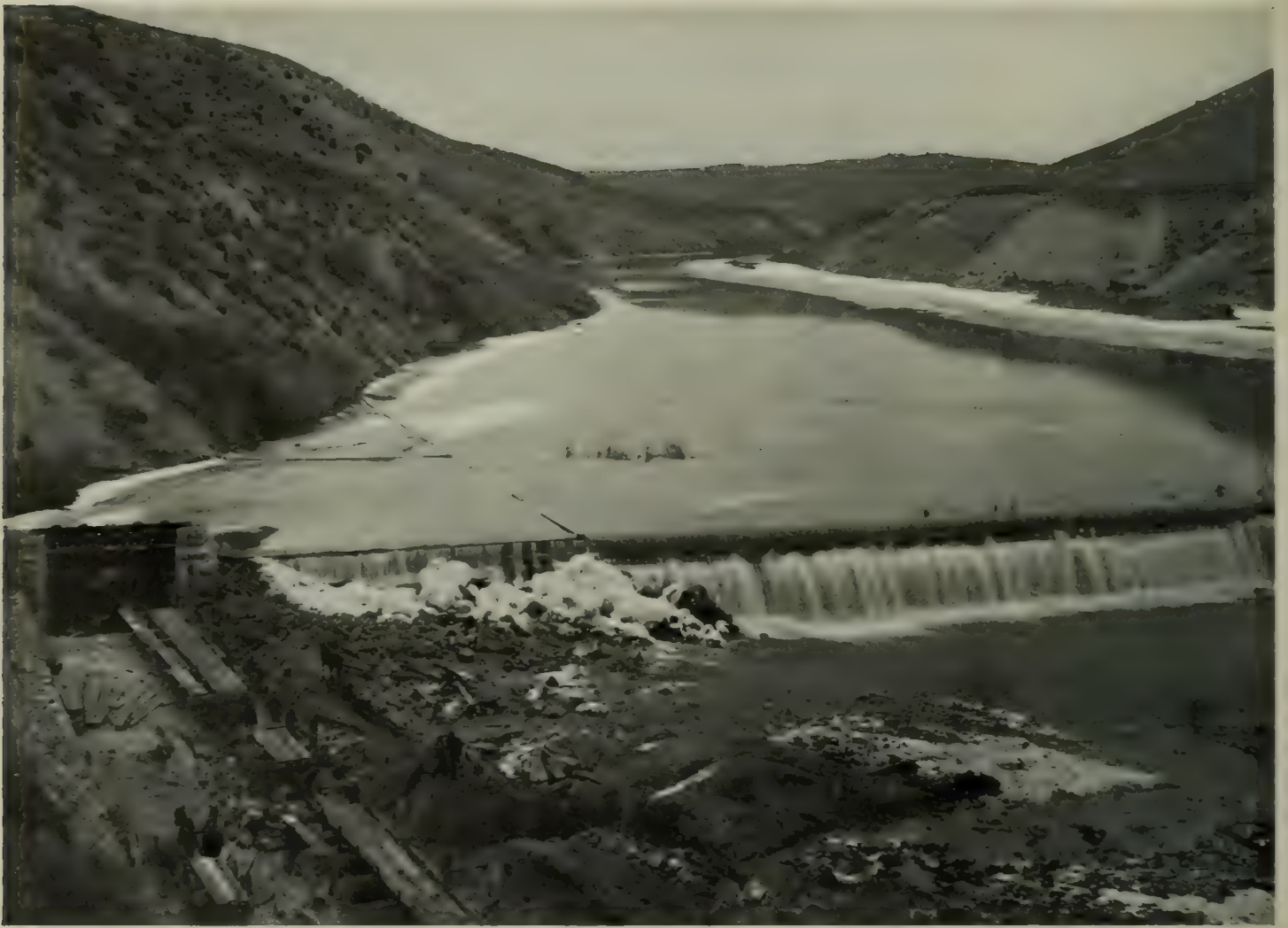
THE BEAR RIVER DAM OWNED BY THE UTAH SUGAR COMPANY
