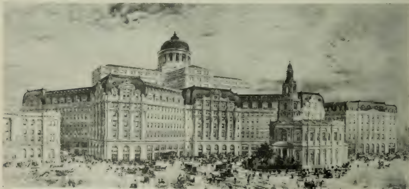
THE FIRST AMERICAN STEEL FRAME STRUCTURE IN LONDON Now building in the Strand
