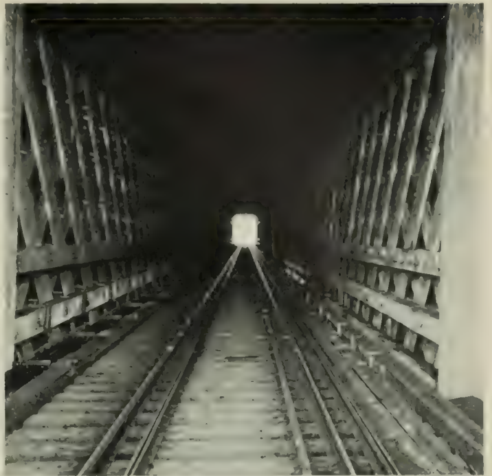
A NEW BRIDGE, SHOWING HEAVY RAILROAD EQUIPMENT
