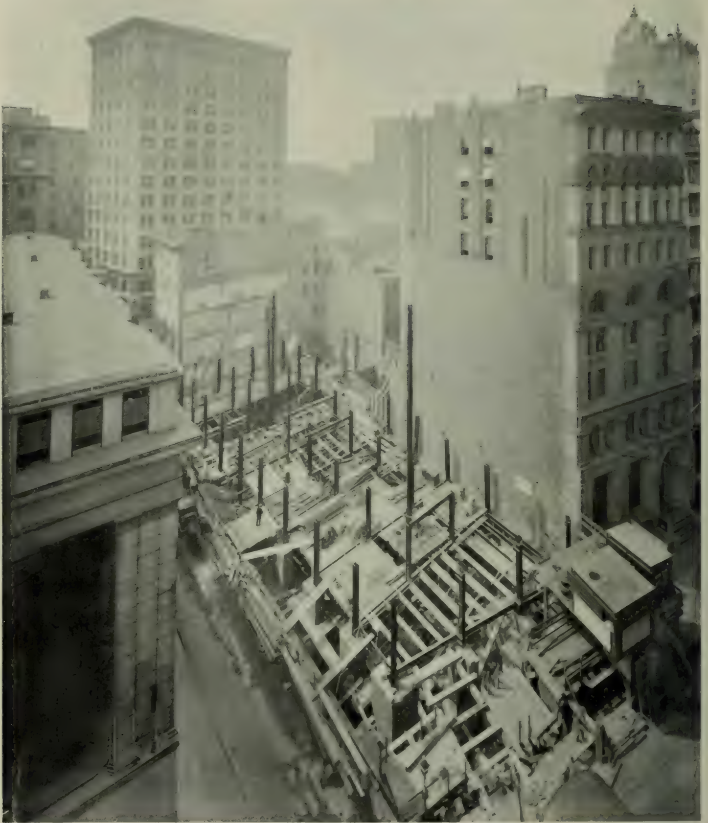
THE FRAMEWORK BEGINNING TO RISE
