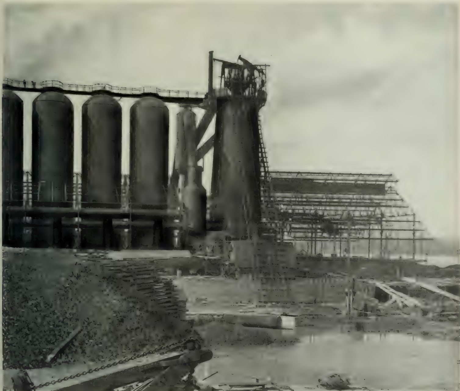
STEEL WORKS AT SYDNEY, NOVA SCOTIA
