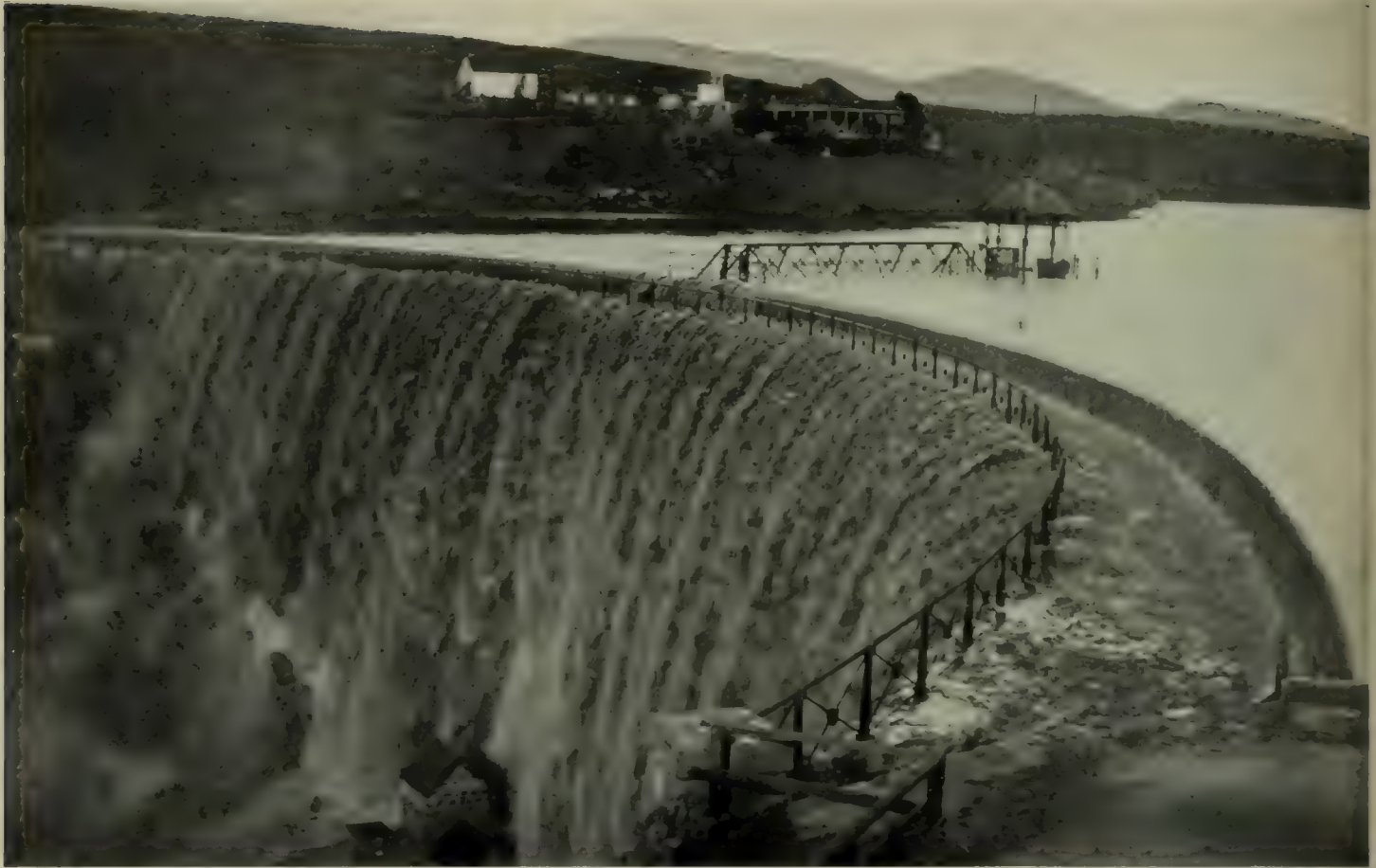
A RESERVOIR OVERFLOWING DURING A HEAVY RAIN, WASTING MILLIONS OF GALLONS OF WATER
