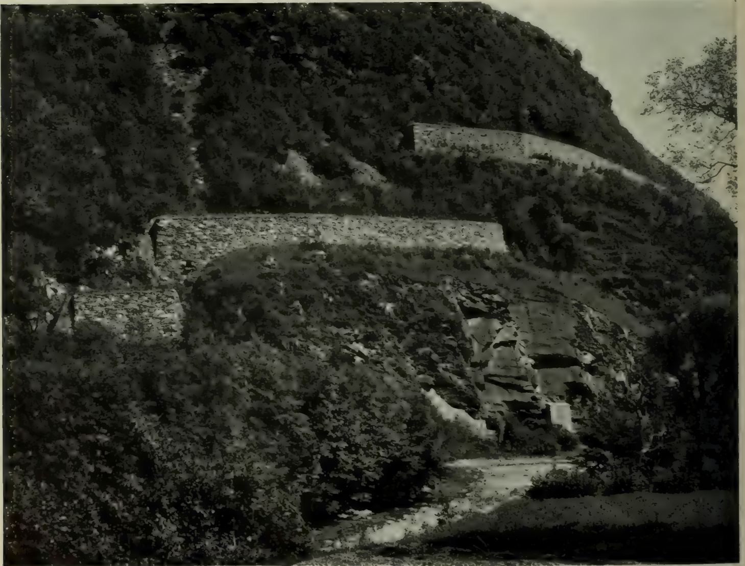
A EUROPEAN HILLSIDE WHERE LANDSLIDES ARE PREVENTED BY BOTH MASONRY AND PINE GROWTH
