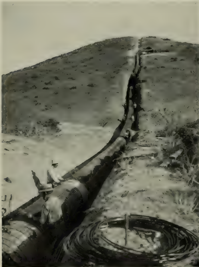
PUTTING THE IRON BANDS ABOUT THE WATER-PIPE LEADING DOWN THE MOUNTAINS
