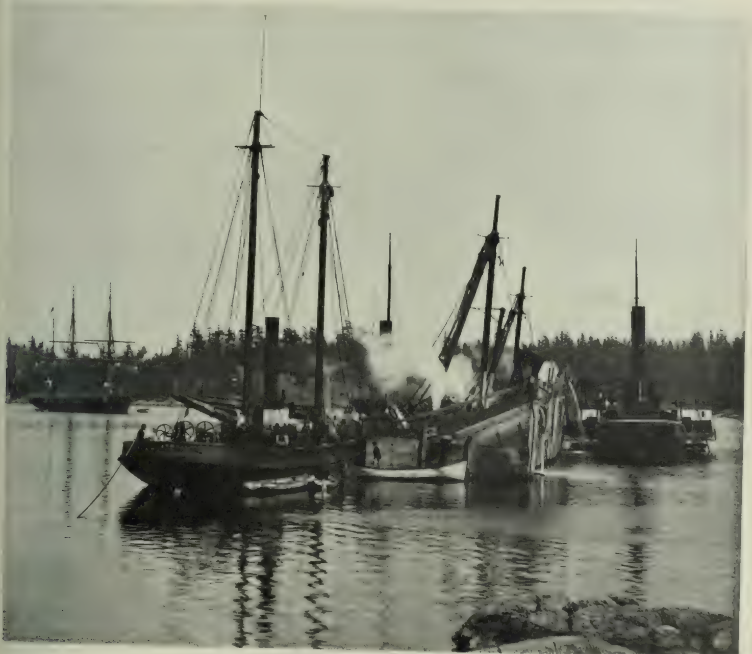
WRECKERS RAISING THE UMATILLA Showing the cofferdam at work
