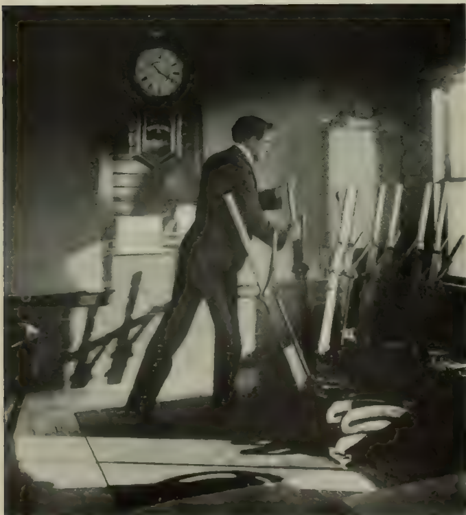
SETTING THE SWITCHES AND SEMAPHORES FROM THE SIGNAL TOWER
