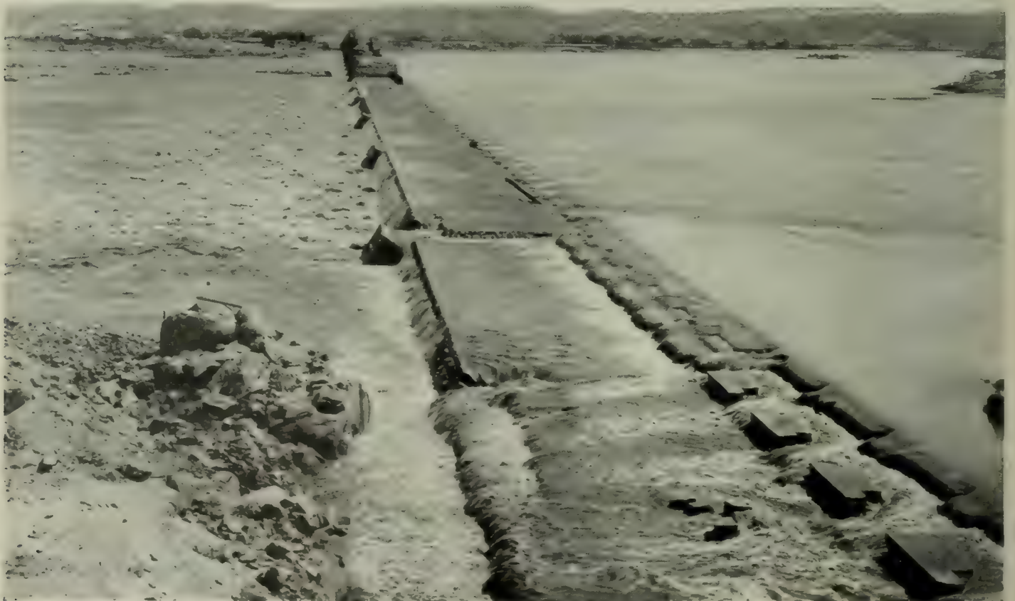
THE DAM HALF BUILT
